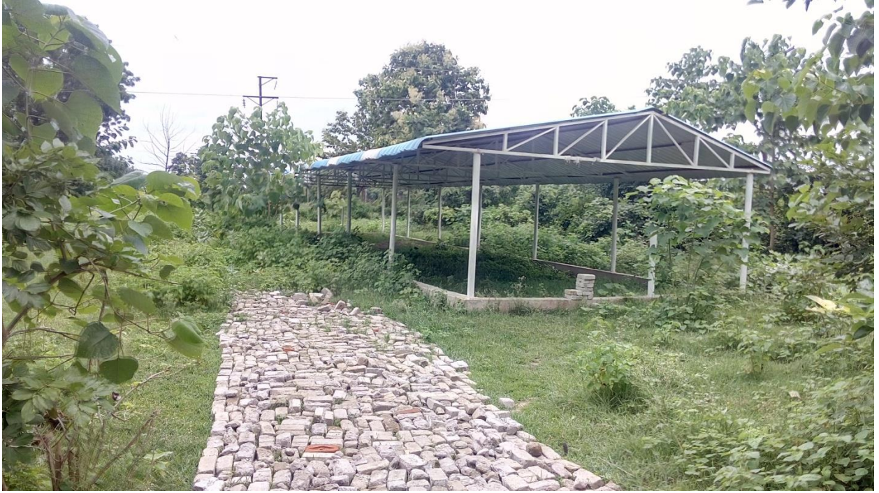
Greenery around newly constructed cycle stand area
